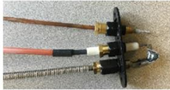
Pilot Mechanism Re-assembled
